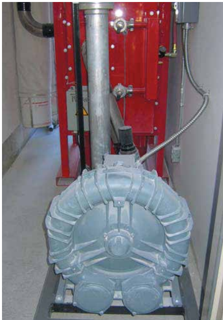
Left: VPK Vacuum Producer as part of a compact central vacuum system, complete with FA 2000 Filtration System. System is so compact, it fit into our customer's closet!
