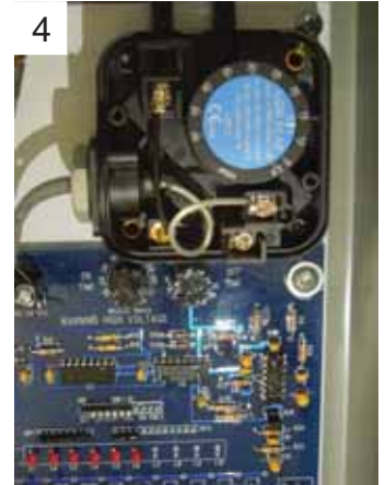
4 Remove the pressure switch snap-on cover from the Dungs conduit enclosure by loosening it's retaining screw and pulling firmly on the bottom end.
