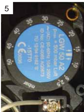
5 Set the Dungs conduit to 14 mbar / 5.6" H 2 O". (Note: 2.49 mbar = 1 H 2 O".)
